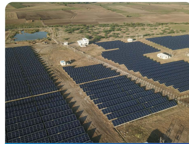
Ground Mount Project
