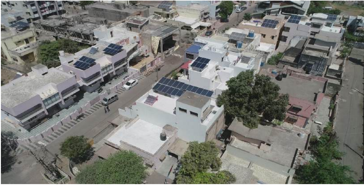
Residential Rooftop Projects
