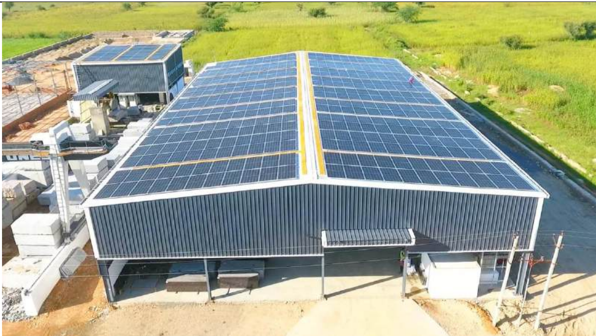
Commercial & Industrial Projects
